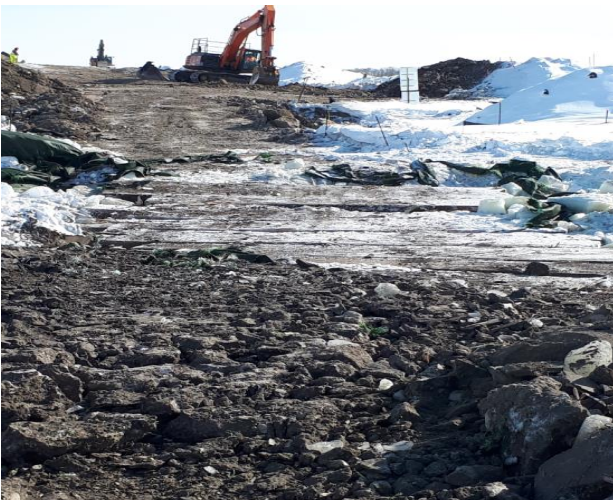
716 + 700 Removing ramp at Montgomery Creek SK WC 79.
