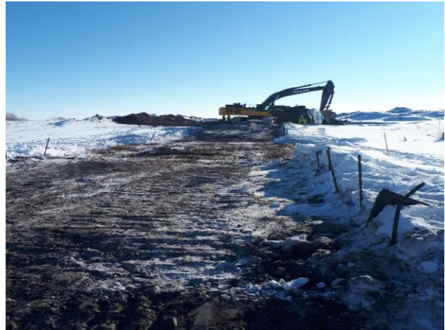
715 + 100 Track hoe stripping wetland SK 752 - WC 78.
