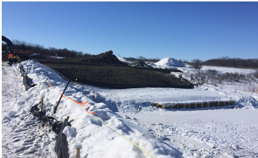
West bank at the Pipestone Creek MB 1010
