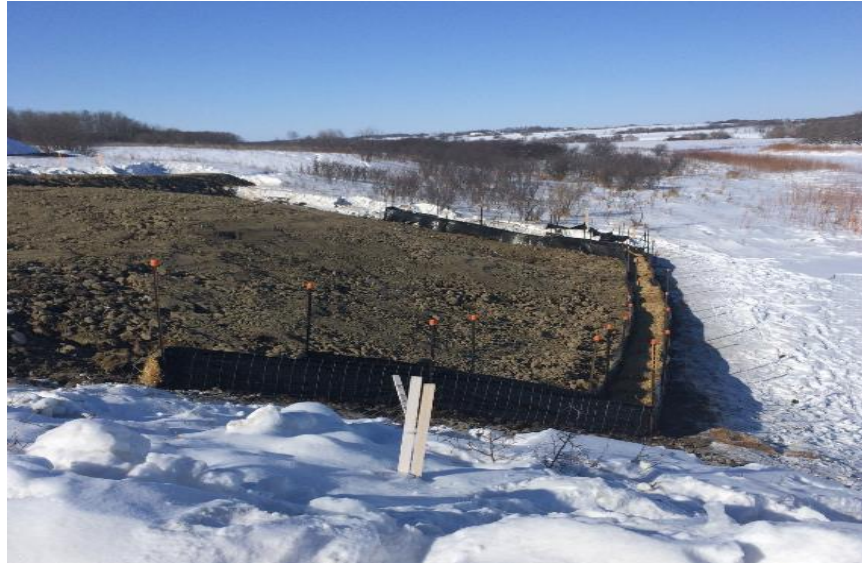
805 + 700 West bank of the Pipestone Creek erosion control.
